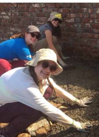
Bethany (foreground) works on building a new classroom
